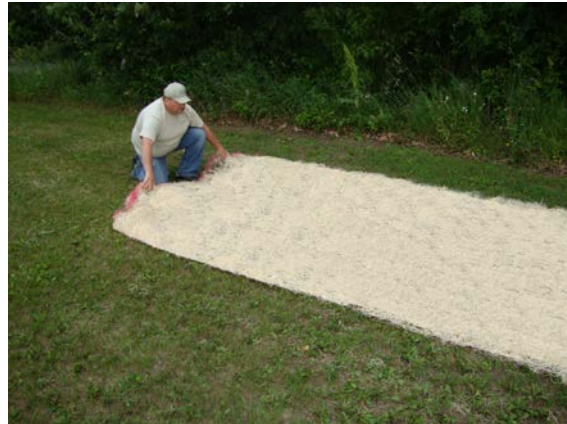
Figure 4. Properly position unrolled RECP for installation.
