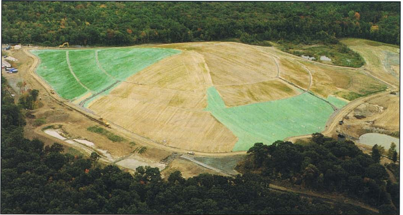
Aerial view of erosion control measures on Laurel Park Landfill.
